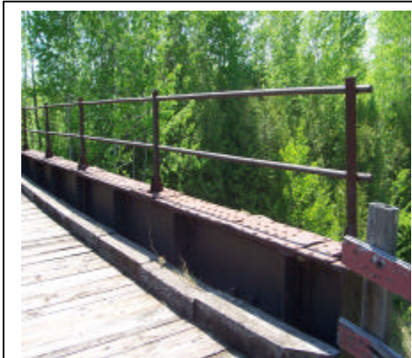
Fig 1: Wrought iron railing
