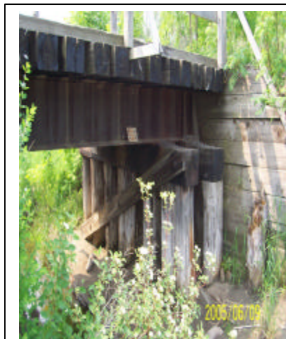
Fig 1: Supporting steel beam and logs
