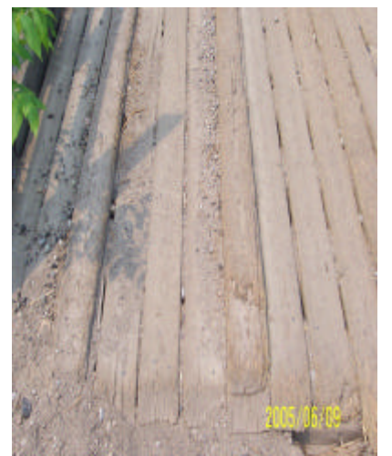
Fig 3: Timber covering the bridge
