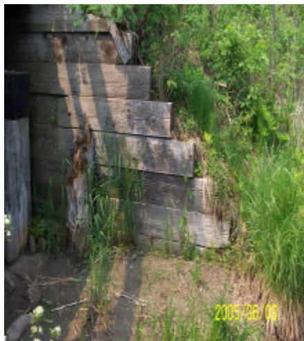
Fig 2: Supporting beams 8x8
