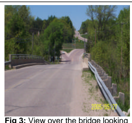
Fig 3: View over the bridge looking north towards Hwy 12
