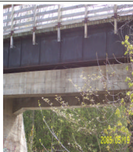
Fig 2: cement and steel support underneath
