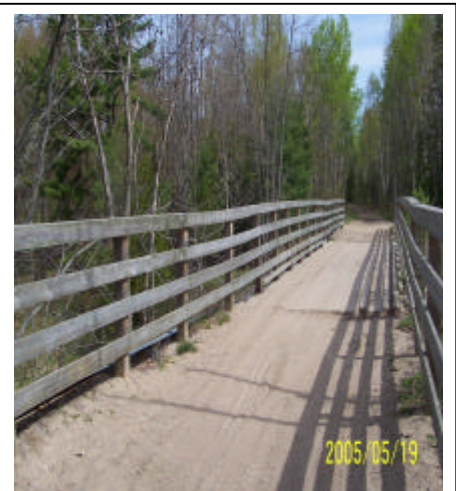
Fig 3: Railings on side put on after for protection of pedestrians
