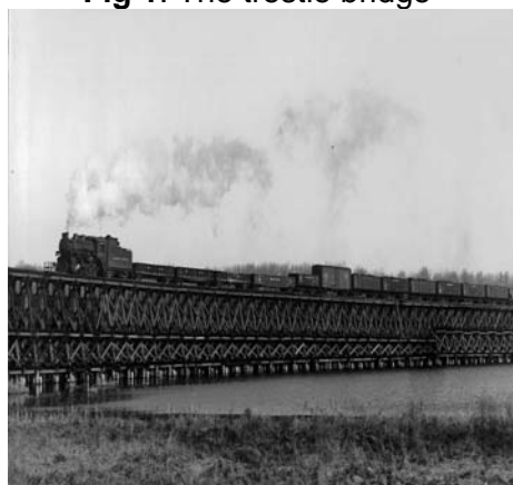
Fig 1: The trestle bridge
