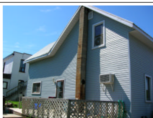
Fig 2: Rear view with cement blocks covering the bricks
